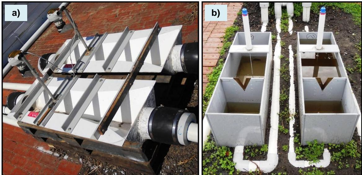
**Figure 2.9: The flumes (a) and overflow pits (b) of the two raingardens. During the monitoring period, the flumes and pits were fitted with waterproof covers (not pictured).**
