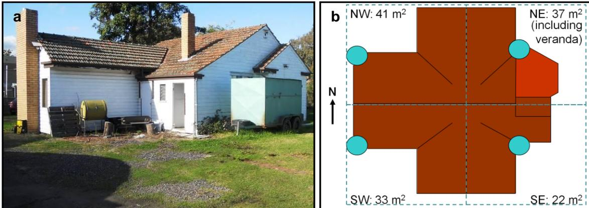
**Figure 2.1:** a) Building 909 in June 2011, viewed from the northwest, prior to construction of the vegetable garden beds, and b) Plan view of the Building 909 roof, showing the positions of the four downpipes (blue circles) and their approximate catchment areas (NW, NE, SW, SE). These downpipes were modified to collectively feed into a splitter box on the northwest side of the house.
