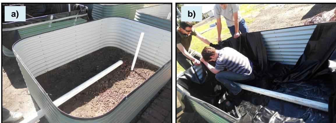
Figure 2.5: The slotted pipe (inlet for roof-water) being installed in the Unlined raingarden (a) and Lined raingarden (b). The pipe was inserted through a hole that was made in the base of the western wall of the bed.
