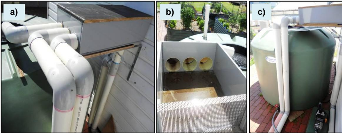
**Figure 2.7: An external (a) and internal (b) view of the splitter box, and its position on top of the rainwater tank (c).**
